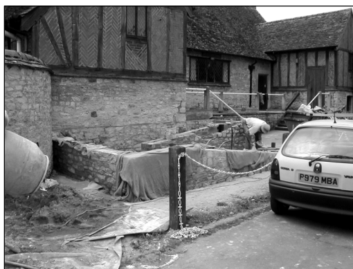
One of the Bernard Hall's other improvements - the disabled ramp being built six years ago.
